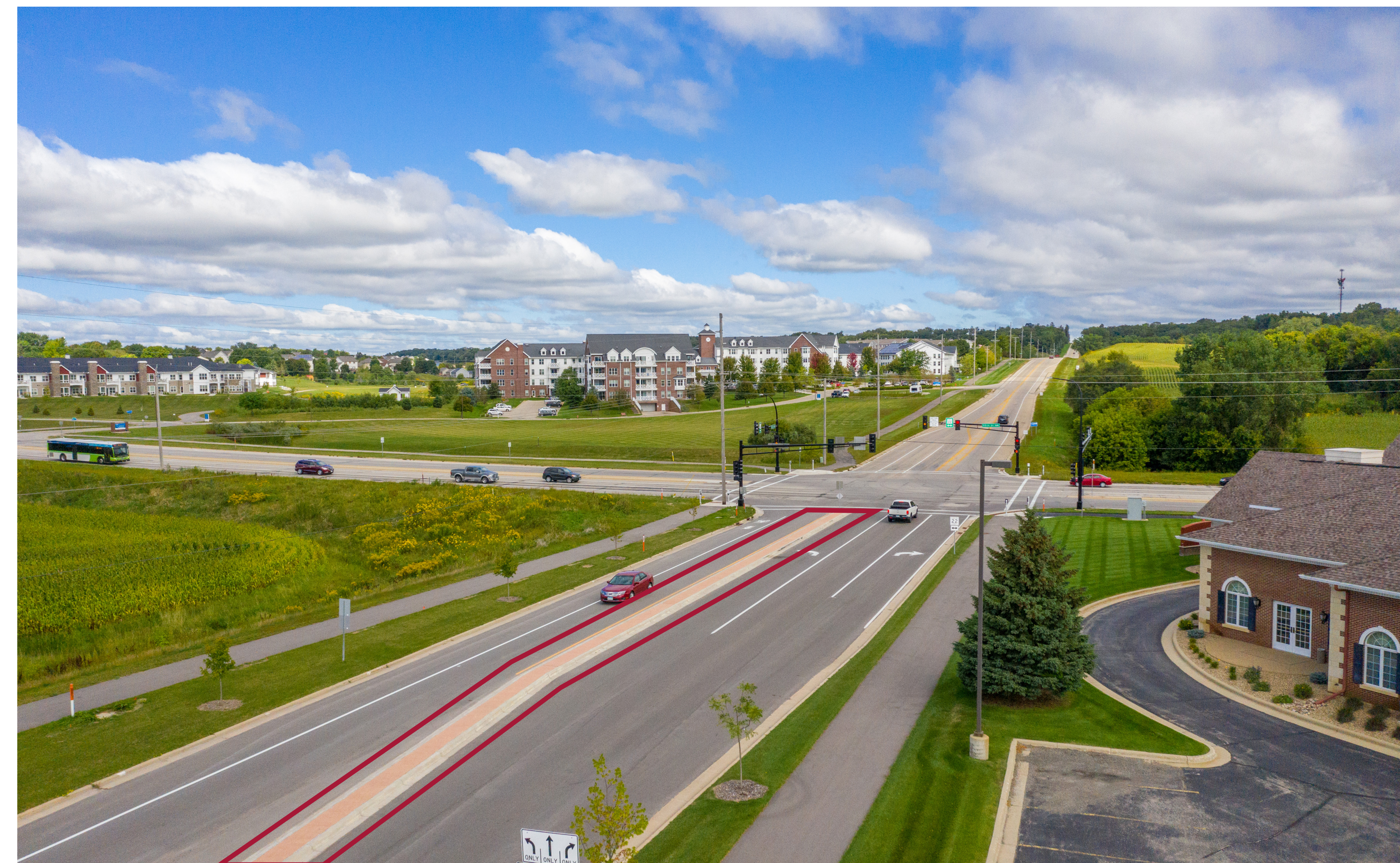
Figure 1: Example of a concrete median in Rochester, MN
